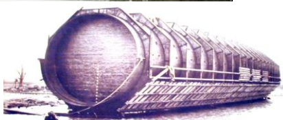
Detroit vehicle tunnel floated to position then sunk 22 feet high
